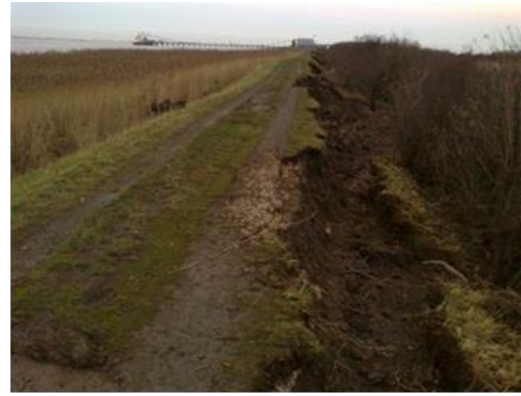
Impacts of December 2013 tidal surge. (left) Barton Haven (right) embankment erosion near New Holland.
