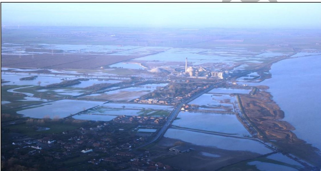
Figure 2 Flooding at South Ferriby and Winteringham Ings, December 2013
