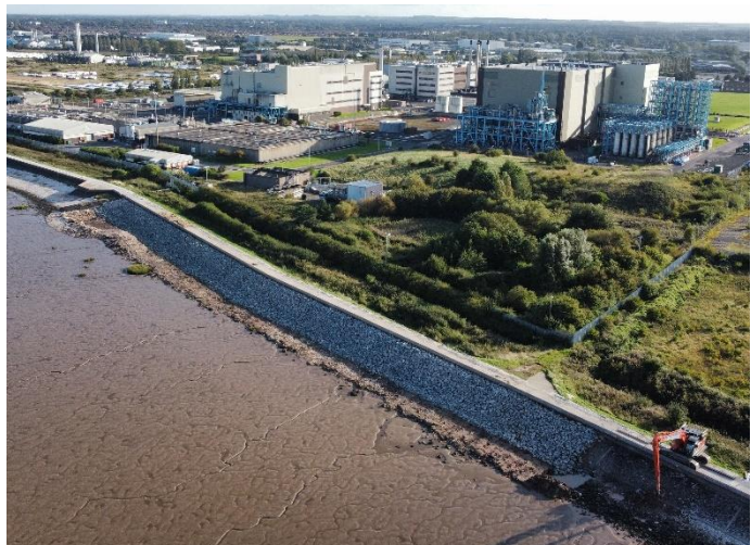
Small rock armour placement
