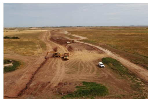
Toe drain excavation and embankment construction in east scheme
