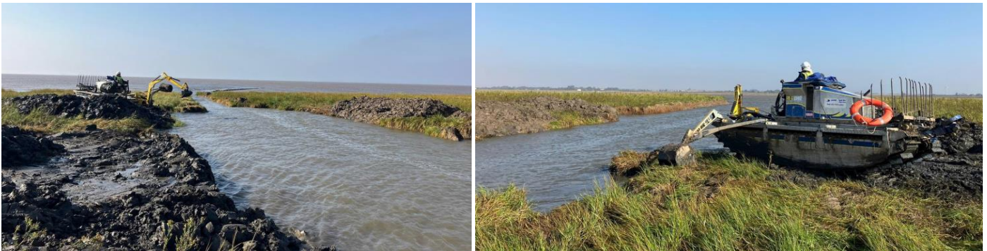
Truxor widening trench on saltmarsh
