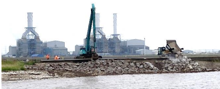
Rock armour installation
