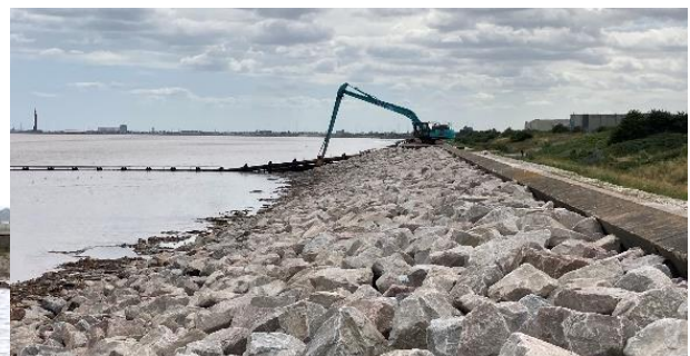
Rock armour placement underway
