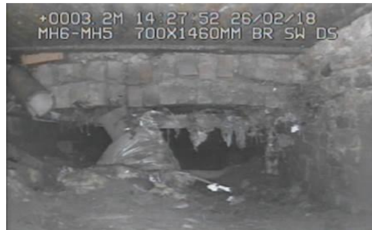
CCTV image of the Vale Brook Culvert
