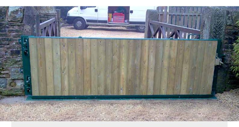
Flood Gates are easy to maintain and can be easily operated by one person, thus representing a quick deployment option.
