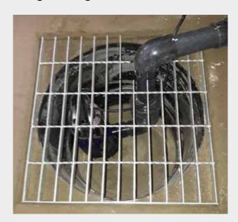
The submersible pump system is installed below ground to a bespoke sump. The pump has an integrated float switch which enables it to automatically switch itself on in the event of rising water, pumping water out and away from the premises.
