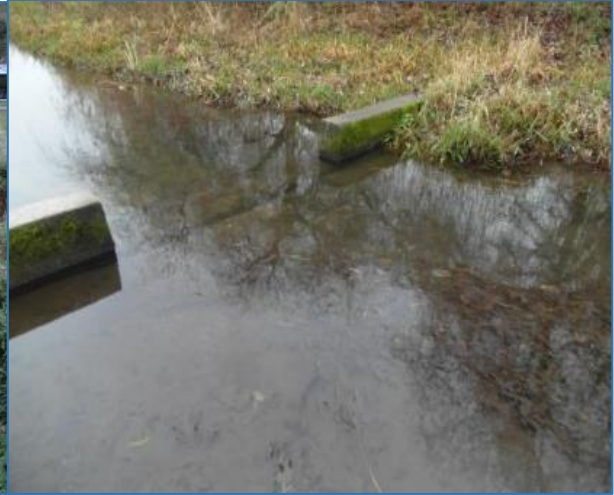
Remains of old weirs, and evidence of siltation on river bed
