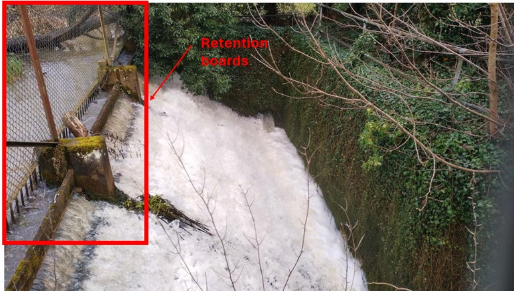
Image showing flood weir and where retention boards were inserted (red box) during periods of low flow.
