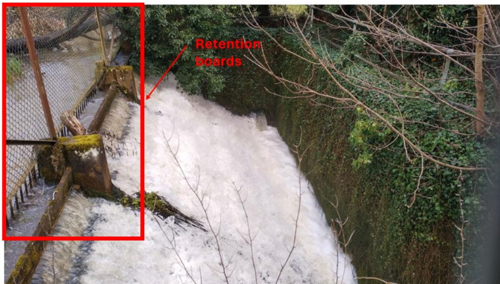
Image showing flood weir and where retention boards are currently inserted (red box) during periods of low flow.
