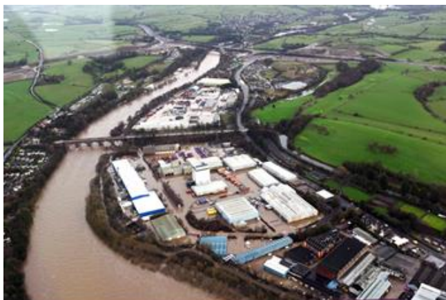
Flooding at Caton Road, Lancaster, December 2015
