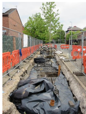
Installation of SuDS enabled tree trench, Salford
