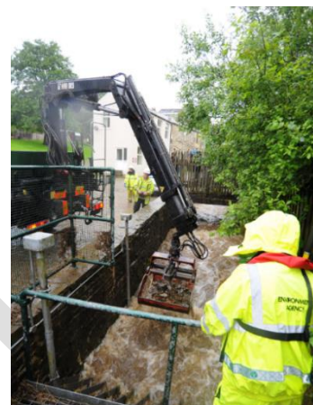
Clearing debris from river screen, Crawshawbooth
