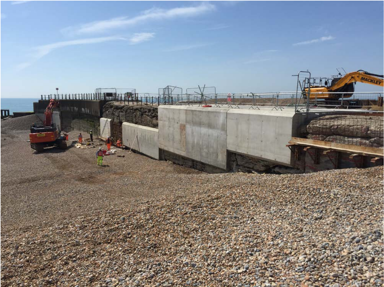
Figure 5: Hastings Coastal Defence Works, Stage 2
