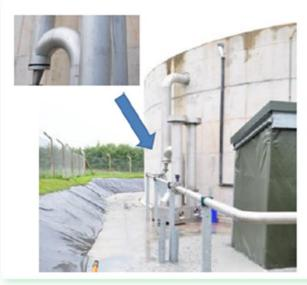
Overflow to PRV very close to reduced size gas pipe. Any foam will quickly enter the PRV
