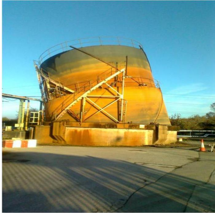
Three sets of guide wheels on the holder had disengaged, its limit switches had failed and sections of the guide rails were corroded. This led to the holder tilting dangerously and gas being released. The Fire Service had to be called because there was a risk of an explosion.
