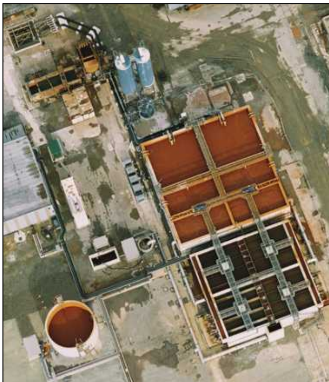
Figure 11. Wheal Jane chemical treatment plant (top photo) and tailings pond used to dispose of the treatment sludge (lower photo)
