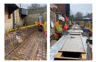
Construction of the flood wall is almost complete. Over 200m3 of concrete has been poured, with approximately 8 tonnes of steel reinforcement. Works on the stone
