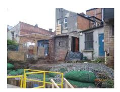
We've also safely removed the structurally unsound outbuilding that was located to the rear of businesses on Crown Square. This has opened up more space and enabled the project team to build a temporary flood defence to plug the gap in the defence line. This temporary defence is made from legato blocks and will now remain in place until the flood wall is completed. The Jackson Civil Engineering team will also be on standby over the festive period should Matlock experience flooding.
