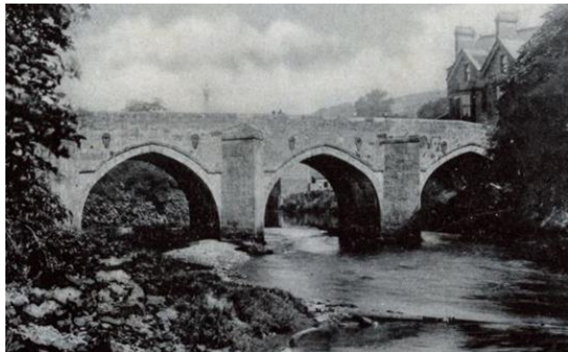
Matlock Bridge in 1903 before widening.
