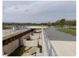
The fish pass is now over 90% complete, with all major works finished. Minor works remain to fit a final supporting beam to the radial gate, after which the pass can be opened to allow full commissioning.
