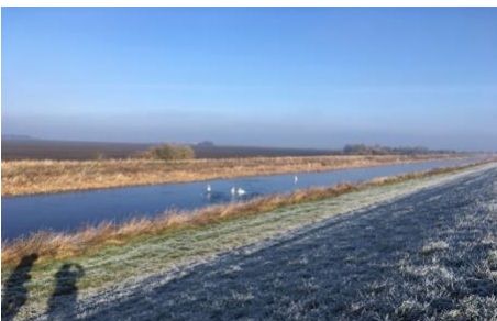
Winter inspection at Welney
