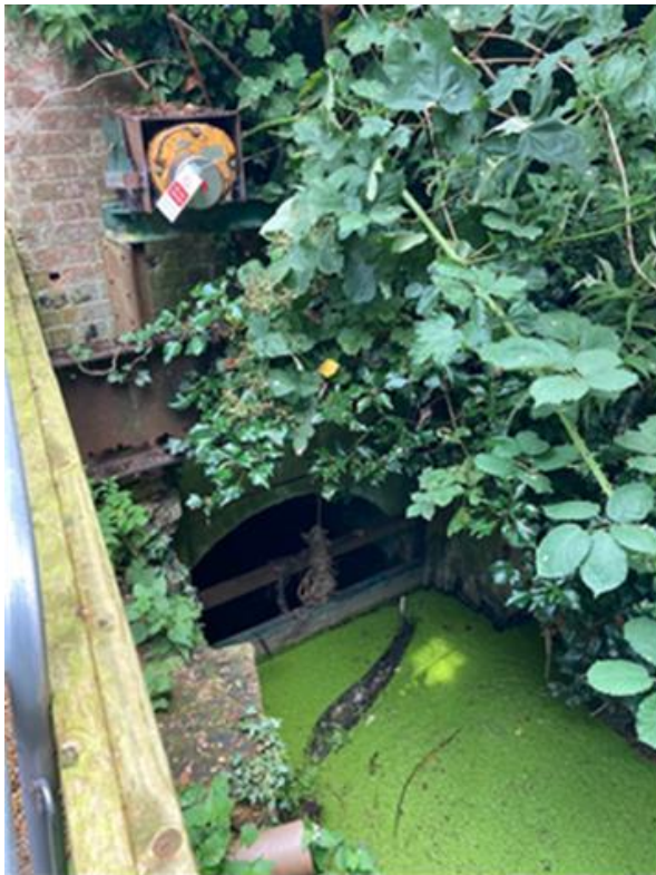
Photograph 1: Environment Agency owned and maintained mill sluice at Wainford Mill.
