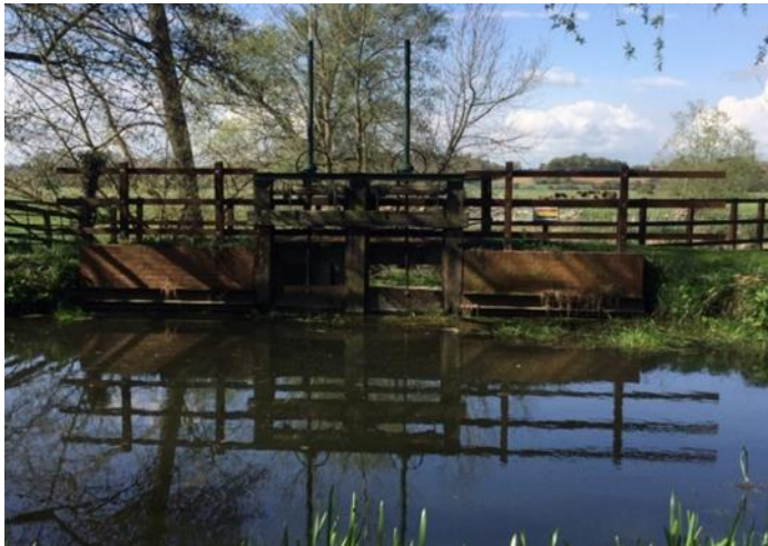
Photograph 1: Environment Agency owned and maintained Hoxne Mill Sluice.
