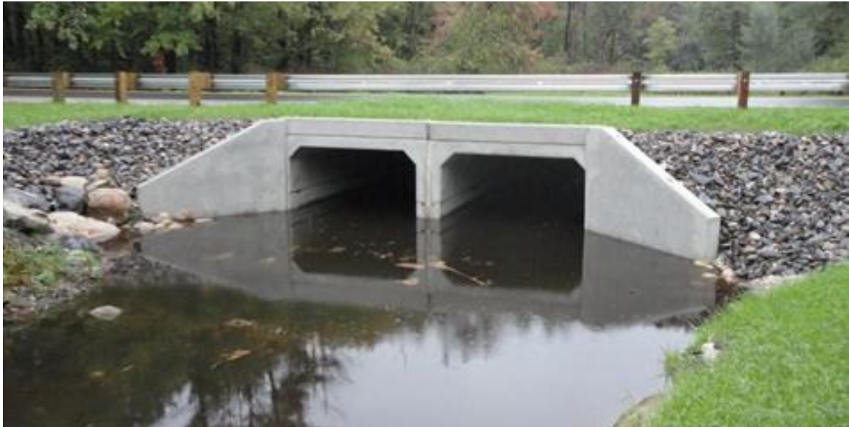
Image showing an example of twin box culvert (Source: Northpoint Engineering)
