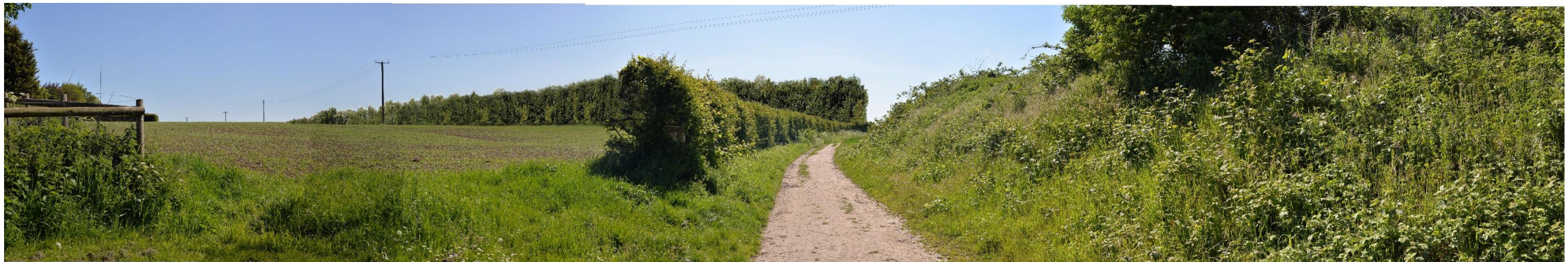
View following restoration and completion of the flood alleviation scheme (15 years following restoration)
