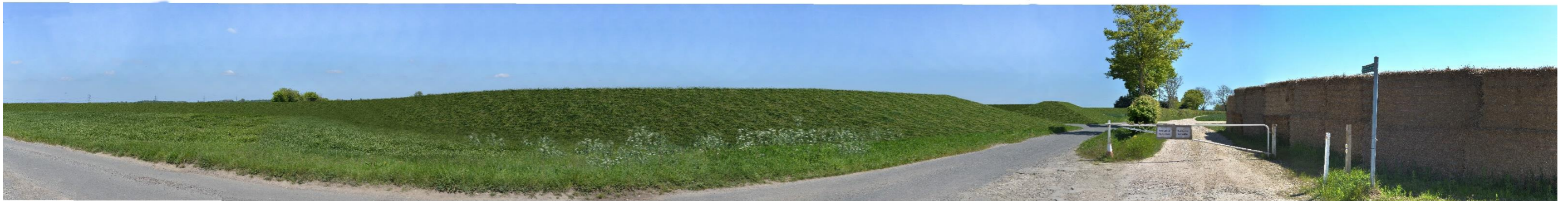
View whilst quarrying, restoration and construction operations progress through Phase A. The bund will screen all Phases of the quarrying and restoration works across the site from Phase A to the completion of Phase D
