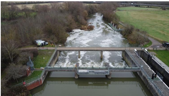
Figure 1: Environment Agency drone photo of sluice. From this perspective the northern bank is on the left-hand side.
