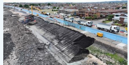
Placing LSA and laying OSA on the revetment at Chapman Sands
