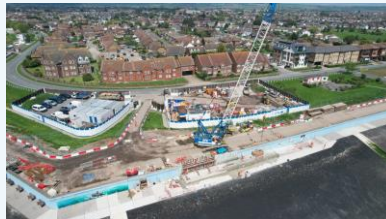
Fisherman's Corner Ramp construction work
