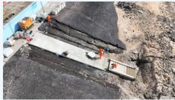
Installation of foreshore steps
