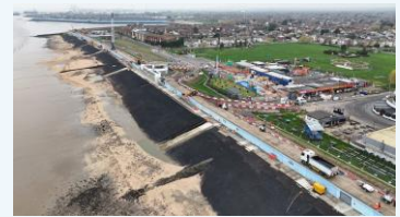
Works on the Labworth frontage
