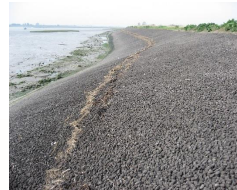
Open Stone Asphalt laid in 2005 at Two Tree Island 2006
