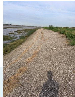
Open Stone Asphalt laid in 2005 at Two Tree Island 2006 2019
