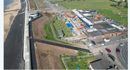
Work at The Labworth
