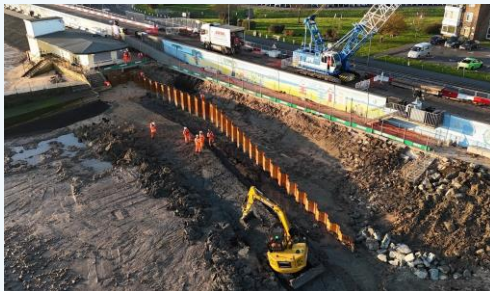
Steel sheet pile wall – Concord Beach
