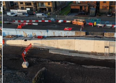
Construction of Chapman Sands access ramp
