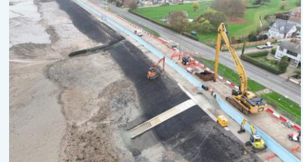
Completed steps and OSA/LSA along Eastern Esplanade
