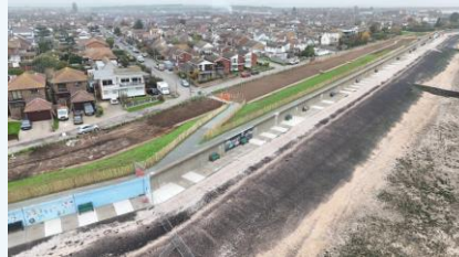
Reinstated/completed area on the landside to Marine Parade
