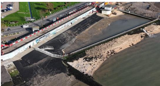
Laying OSA/LSA at the western tidal pool
