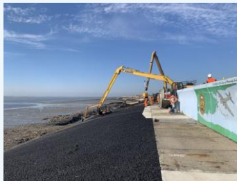
Placing Open Stone Asphalt (OSA) at Leigh Beck
