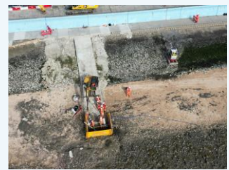
Construction works and seaweed cleaning
