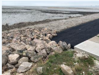
New revetment at Leigh Beck
