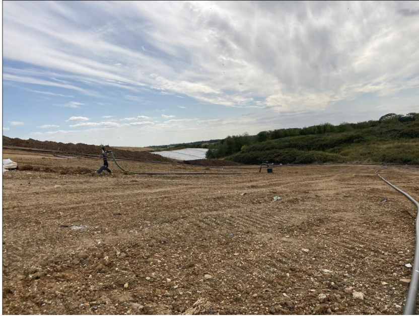
Restoration soils applied (foreground) and area of permanent capping (background)
