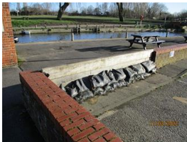
Figure 2 - Access point which could be closed to the east of the Harbour Master's office.
