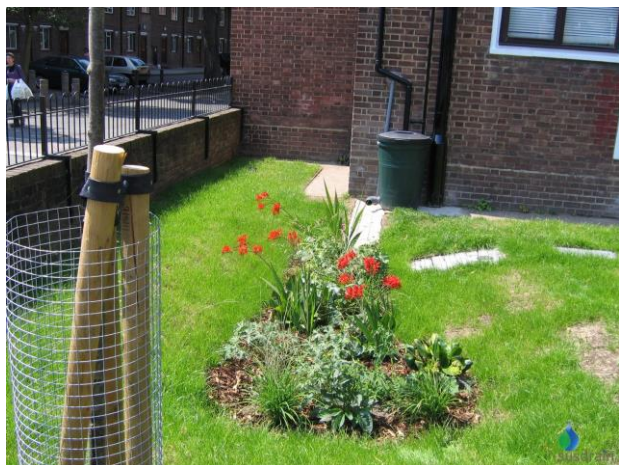
Figure 4 - Example of a sustainable drainage solution in the form of a water but and rain garden
