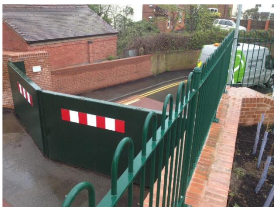
Figure 1 - Example of a flood gate
