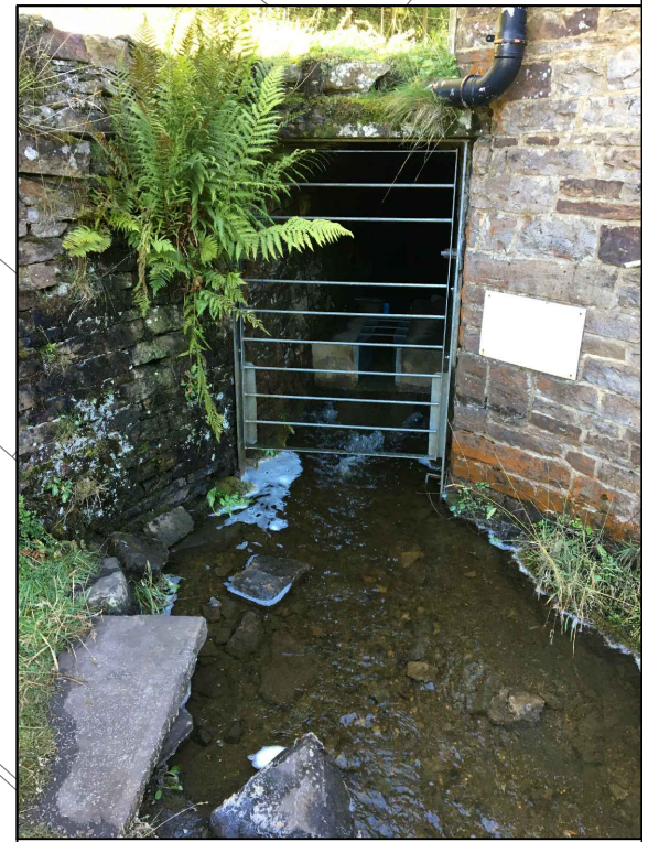
PHOTOGRAPH 2 - RAMPGILL ADIT DISCHARGE
