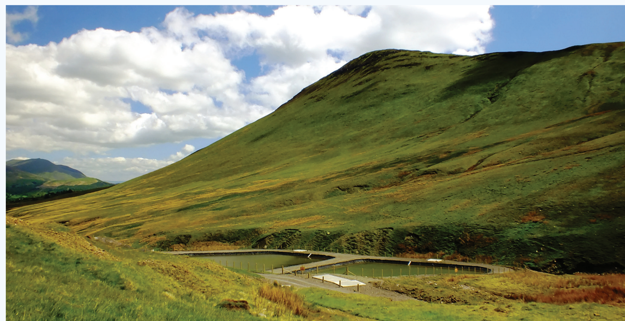
Example of compost-based treatment ponds at Force Crag in the Lake District
