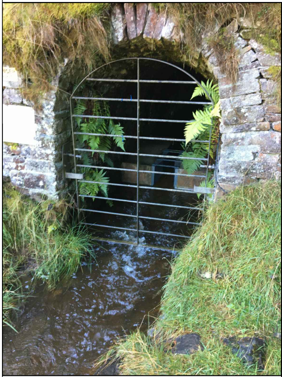
PHOTOGRAPH 1 - CAPLECLEUGH ADIT DISCHARGE
