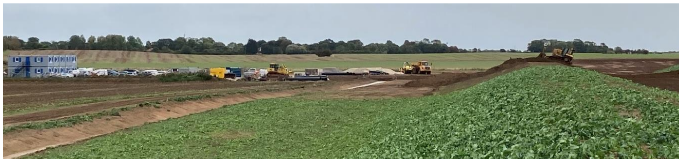
Picture of OtSMRS prior to winter decommissioning
